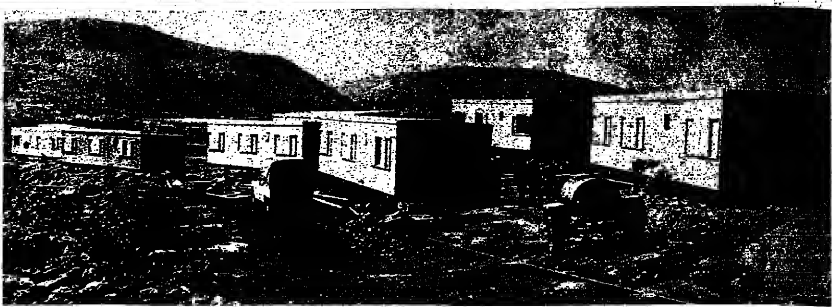
These are the prefabricated houses which the settlers at Eilon Moreh managed to put up before yesterday's court order forbidding all further construction at the site.
